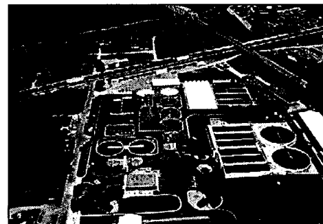
Parkersburg Utility Board's 19th St. WWTP.
