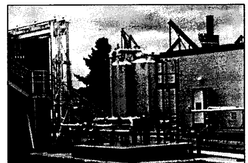
Biological H 2 S scrubbers.
