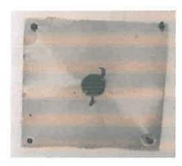
Below is an example of the requested lighting installation in a similarly constructed facility with a similar plaster & wire ceiling. 3/4"x 2'x2' painted plywood patch with silicon or adhesive bead to prevent airflow in and out of attic space.
