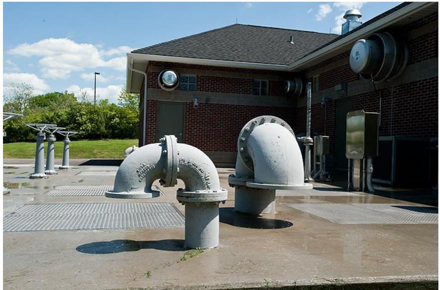
Approximately 40,000 linear feet of 30-inch and 36-inch force main was constructed across the center of Lexington in a combination of private easements and crowded city streets. Several miles of force main were installed parallel to Interstate 75 and inside the interstate's right-of-way. GRW coordinated extensively with local politicians, and state and federal agencies including the Kentucky Transportation Cabinet and the Federal Highway Administration.
