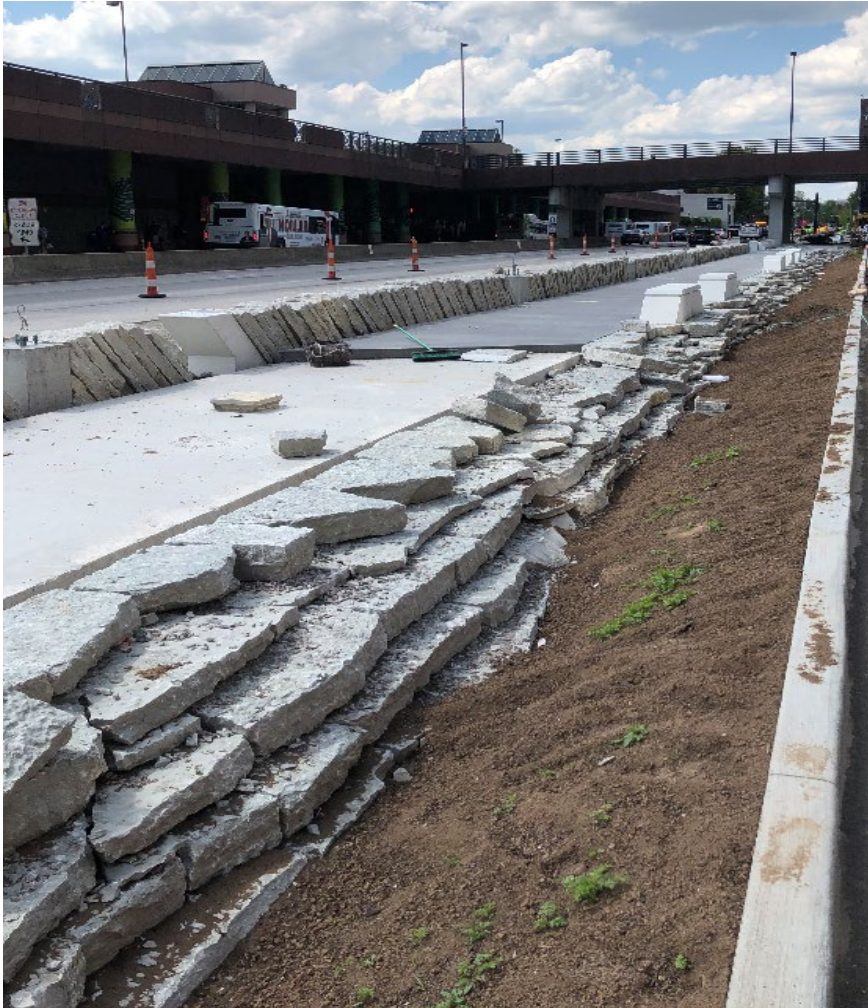
Karst Embankment along Urban Rain Gardens and Bioswales
