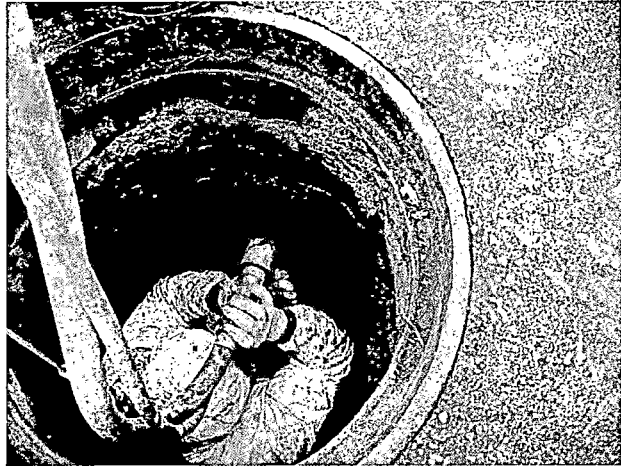
We designed wastewater gravity sewer rehabilitations/replacements to support Nashville Metro's Consent Decree-mandated capital improvement program.
