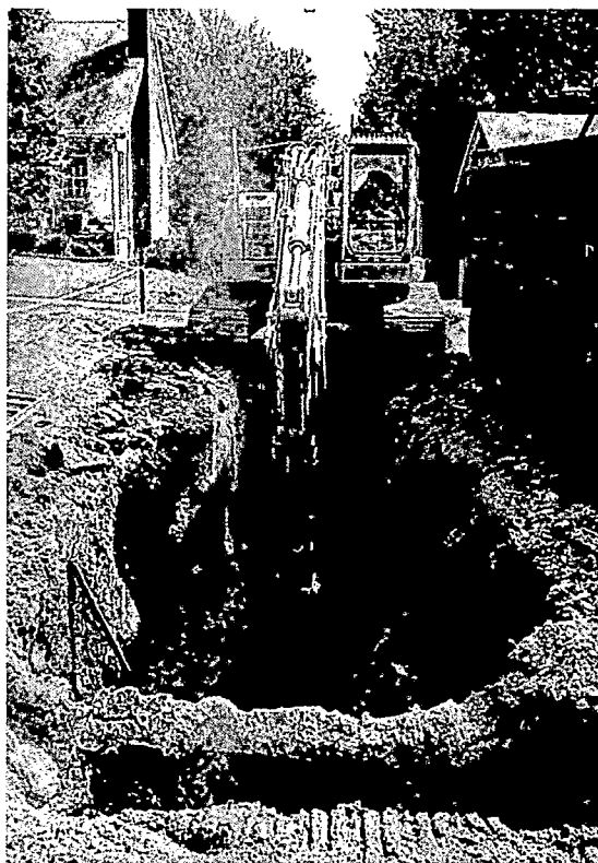
Stantec capitalized on realignment opportunities in the design of the Elkhorn Park trunk sewer replacement to reduce construction costs and minimize disruption to residents in this mature neighborhood.
