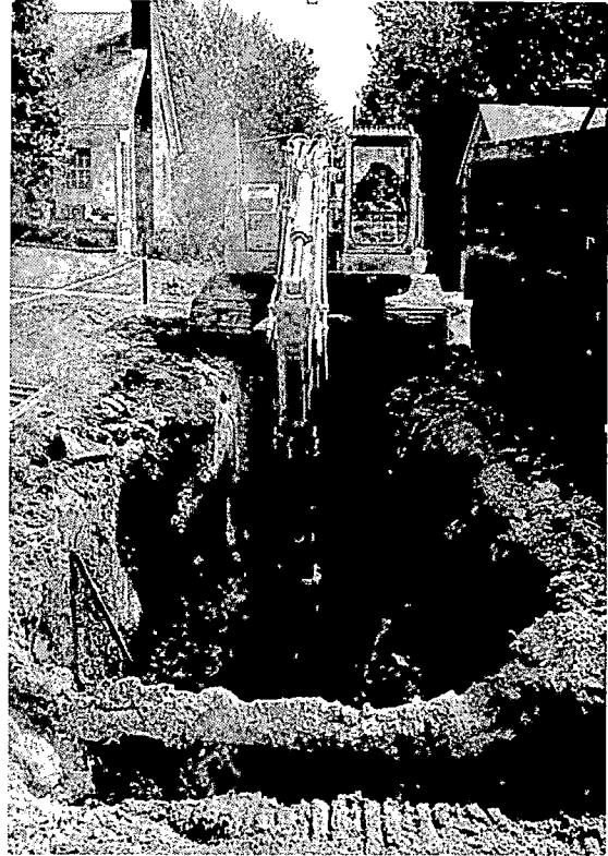
Stantec capitalized on realignment opportunities in the design of the Elkhorn Park trunk sewer replacement to reduce construction costs and minimize disruption to residents in this mature neighborhood.
