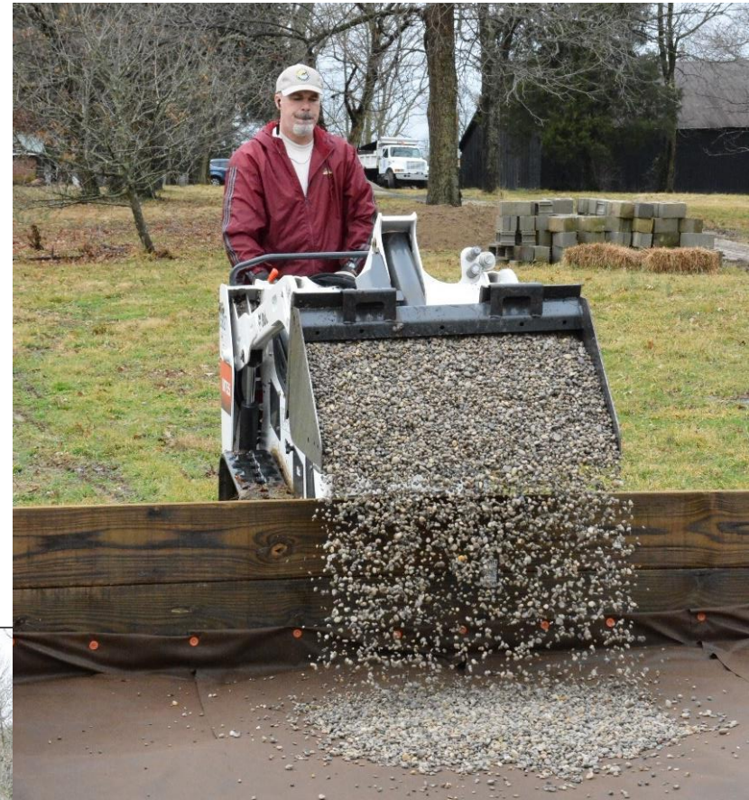
Filling with sand and gravel
