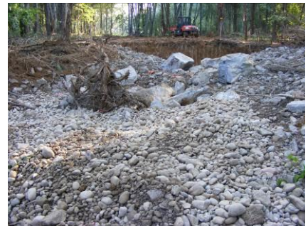
Constructed riffle with spawning gravel.
