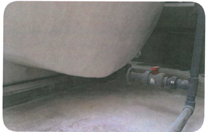
Leak fixed and drain plugged to minimize future leaks
