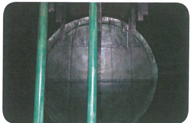
Storage tank interior after repairs and relining
