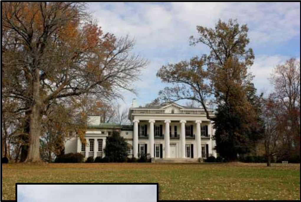
Figure 26. Woodburn (the main residence of the Alexander Estate) on the north side of Old Frankfort Pike in the Big Sink Rural Historic District.
