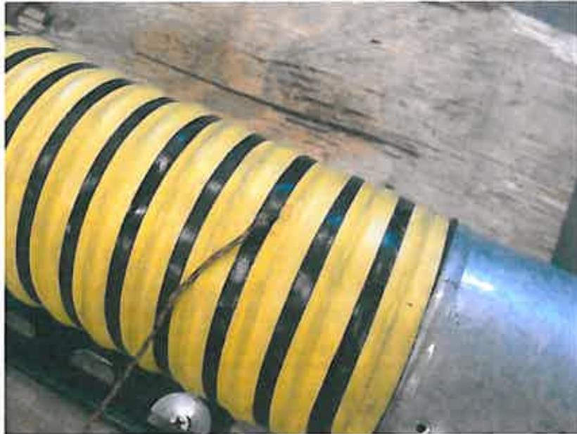
Photo 1 – Attachment of the Hose to the Duct Assembly
