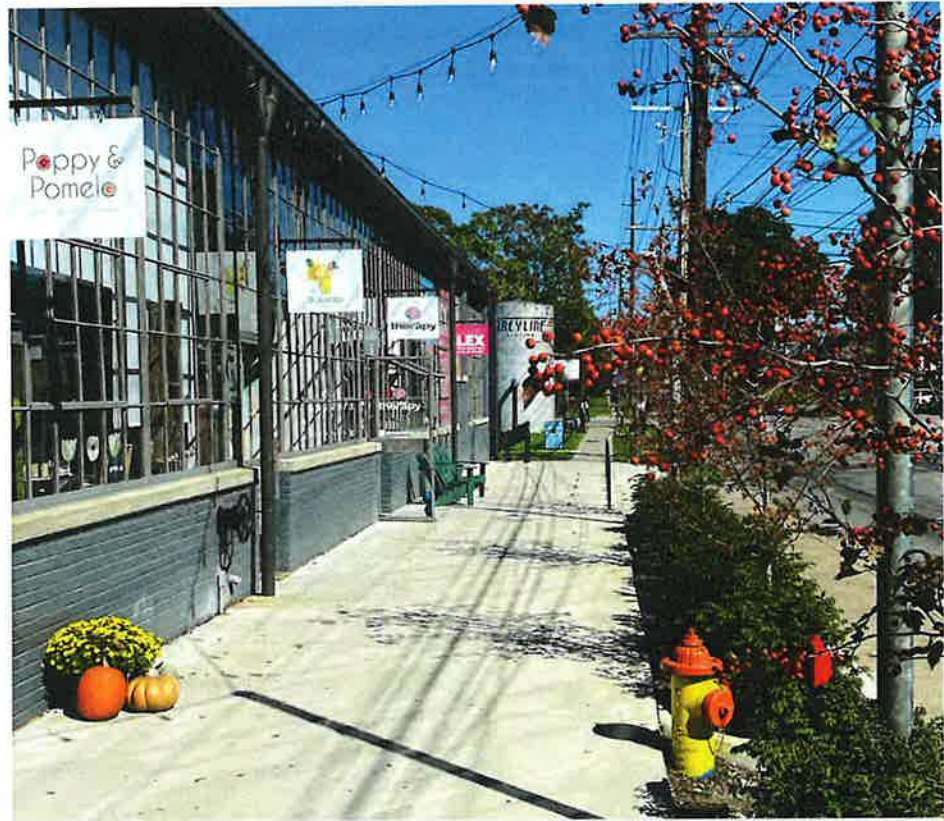
Greyline Station's design balanced public access with stormwater quality features. A divided sidewalk provides a well-balanced mix of store-frontage space, pedestrian through traffic (along North Limestone), and a water quality infiltration strip.
