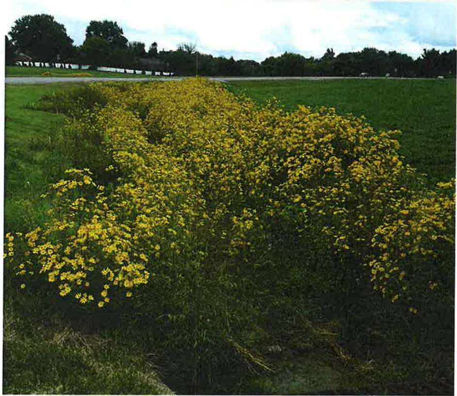
University of Kentucky Alumni Drive BioSwale - completed with a FY2018 LFUCG Stormwater Quality Projects Incentive Grant (completed by Stantec/Ridgewater Design/Build Team). Our Project Team is experienced with the use of native (and colorful) vegetation in our designs.
