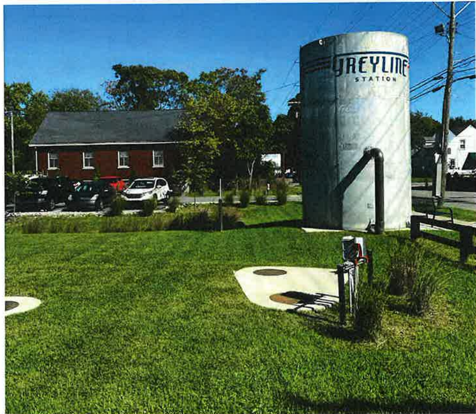
Greylne Station Rainwater Harvest System - completed with a FY2020 LFUCG Stormwater Quality Projects Incentive Grant (Designed/Built by the Stantec/Ridgewater Team). Project was recognized with the 2021 ACEC Grand Award.
