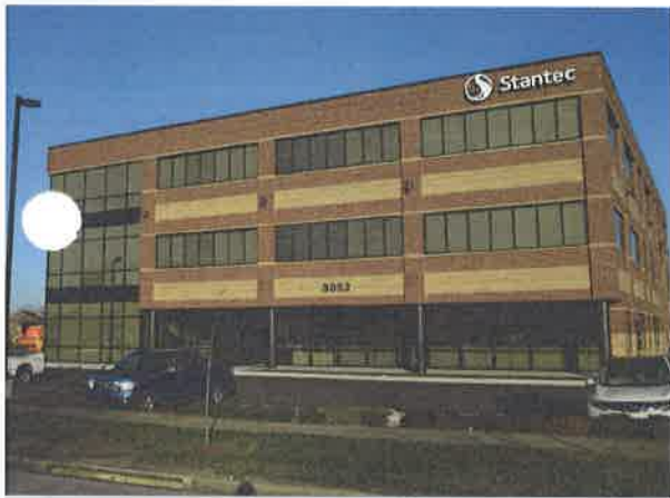
Stantec's Lexington office at 3052 Beaumont Centre Circle
