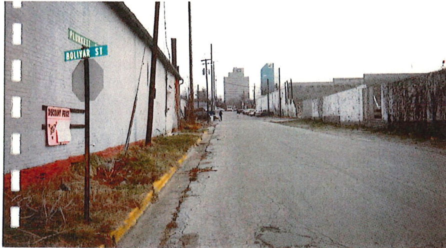
Abandoned warehouse at Plunkett Street and Bolivar Street, looking north (the Properties located on left)
