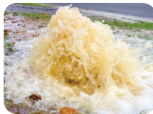
Sanitary sewer overflow
