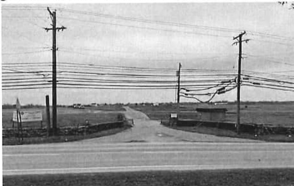
Existing overhead utilities along Old Frankfort Pike.
