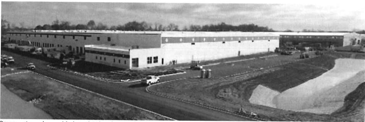
Green wet ponds provided mechanism for site dewatering. (12/8/16)
