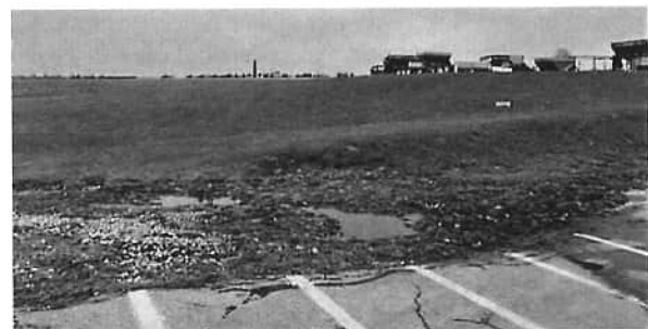
Steep slopes adjacent to existing building pad.
