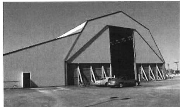
Illinois Tollway's new salt storage facility.
