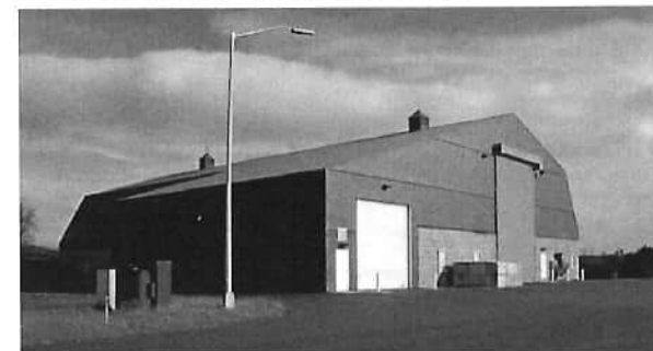
Dane County salt shed designed as part of the Verona Road project.
