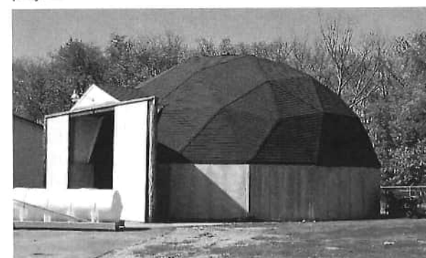
Fontana's salt storage building.
