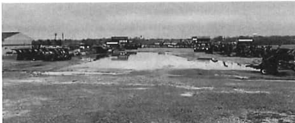
Existing building pad and ponded water.
