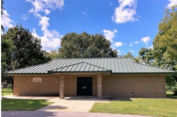
Coolavin Park 550 W. 6 th St. • 40508 1 st District
