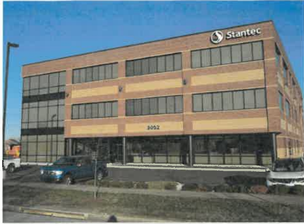
Stantec's Lexington office at 3052 Beaumont Centre Circle
