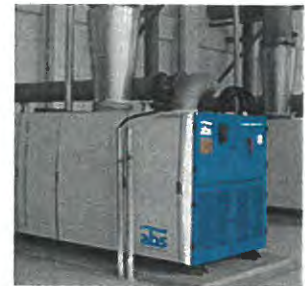
Example of new Sulzer Zone 2 blower (Source Sulzer).
