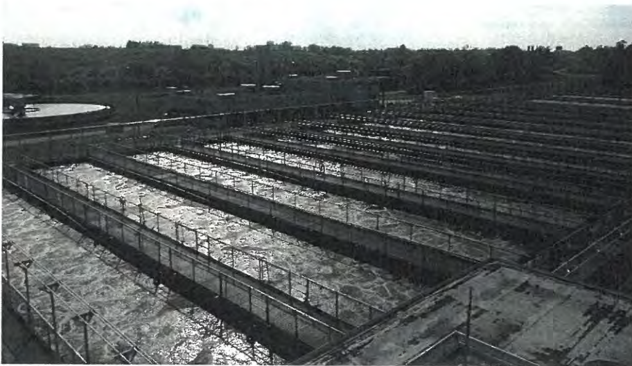
Aeration Tanks at Town Branch WWTP
