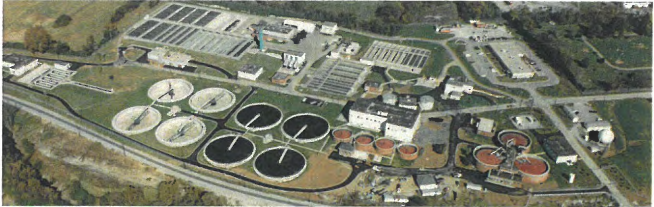
Town Branch Waste Water Treatment Plant.
