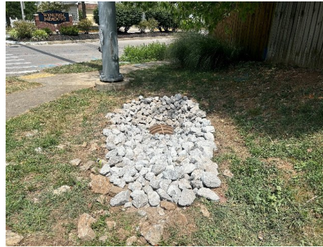
Wyndham Hills & Clays Mills (Buried Inlet – Impacted Storm Pipe)
