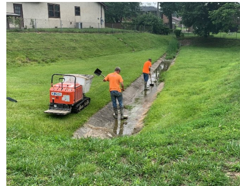
Cleaning Concrete Flumes
