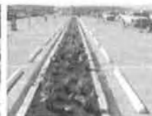
Parking Lot Bioretention
