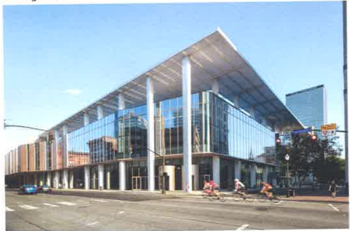
Kentucky International Convention Center Expansion , Louisville, KY
