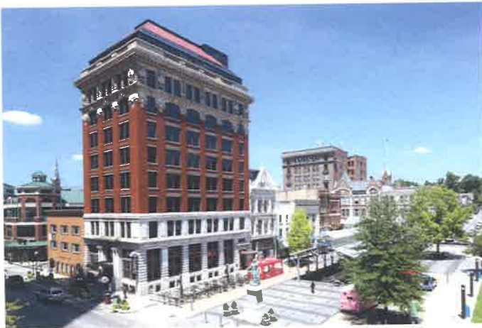
Court Square Building Renovation , Lexington, KY
