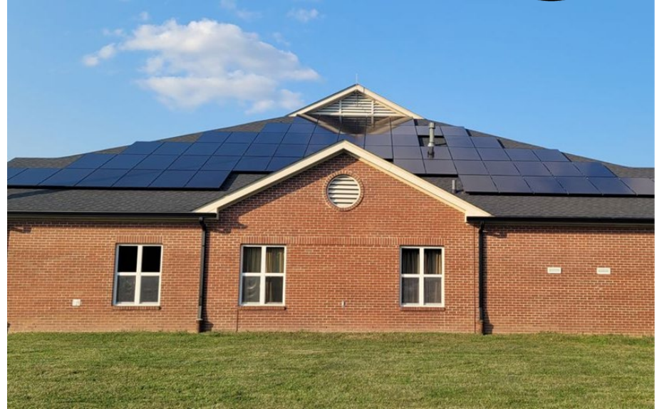
Fire Station 21 in Gleneagles: Proving Solar Viability in Lexington
