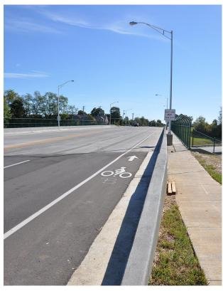
congestion and improves safety and includes typical three-lane urban roadway section with bicycle lanes, sidewalks and handicap ramps; center two-way left turn lane and additional travel lanes and right turn lanes; curb and gutters, and roadway drainage primarily via storm sewers. Included field data collection and survey work. **Client Contact:** Keith Lovan, PE, KYTC Bicycle & Pedestrian Coordinator, (859) 258-3478, keith.lovan@ky.gov
