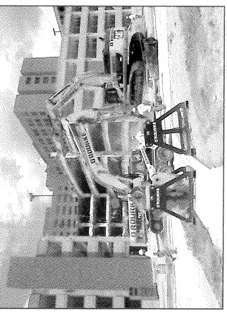
Mass and selective demolition of a 5-story parking garage and ramp that was attached to the main hospital by a common wall. On the other side of this common wall was the hospital's CAT scan machines, linear accelerators & other highly sensitive equipment. Due to the strict vibration restrictions conventional demolition methods could not be utilized. A combination of sawcutting and the use of excavators outfitted with demolition specialty attachments were used.
