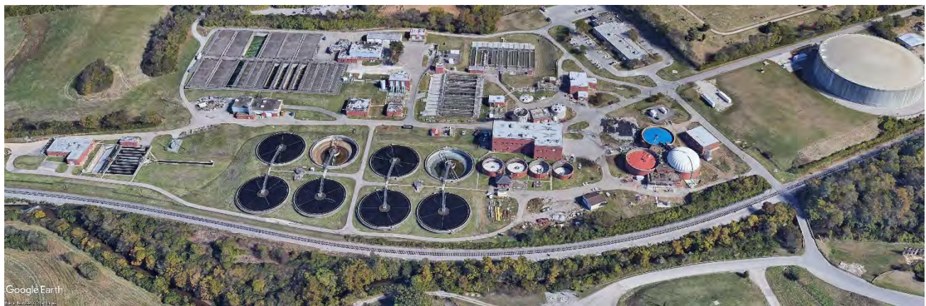
Town Branch Wastewater Treatment Plant.
