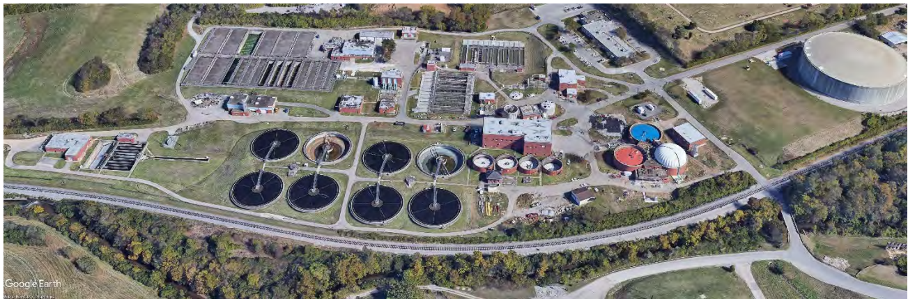
Town Branch Wastewater Treatment Plant.
