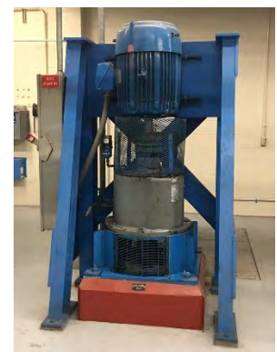
RAS pump motor installation.
