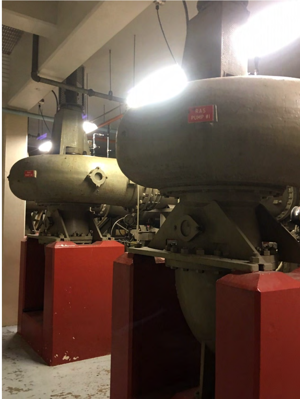
RAS pumps located in lower level.
