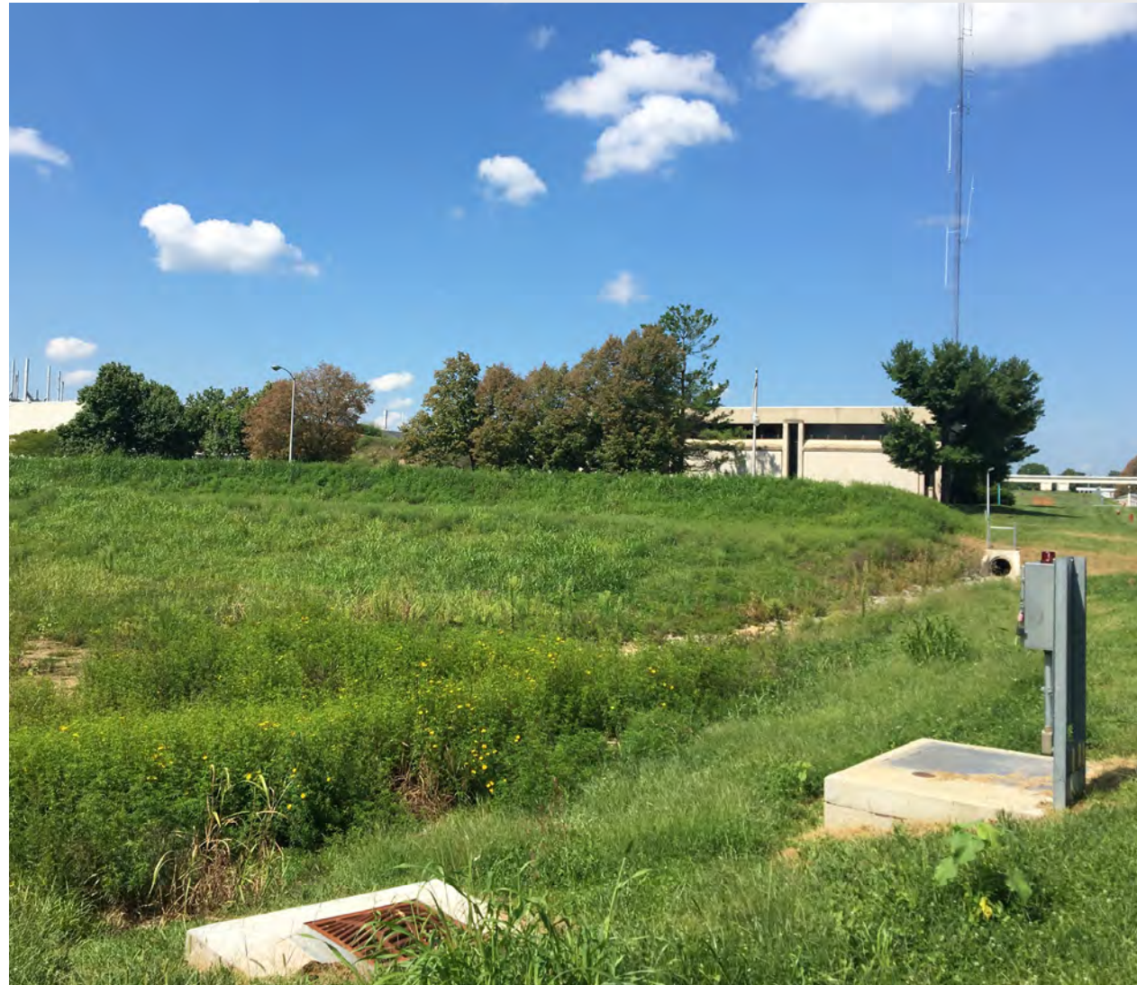
Lexmark Rainwater Harvest System - completed with a FY2013 LFUCG Stormwater Quality Projects Incentive Grant (completed by Stantec/Ridgewater Design/Build Team). Project was recognized with the 2019 ACEC Grand Conceptor Award.
