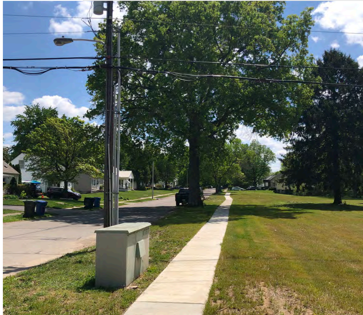
A potential project challenge will be underground/above ground utilities along the Furlong Drive Greenway.
