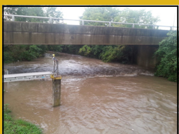
Proposed location of the stream gage and telemetry. Existing VEGA gage along Jimmie Drive. Photo taken during storm event on September 2, 2014.
