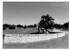
America's Byways®. The new dry stone fence was designed and constructed to mimic an existing dry stone fence found on the property opposite of Old Frankfort Pike. On time and without a single change order, Marrillia completed the construction of approximately 708 linear feet of dry stone fence, construction staking, demolition of existing retaining walls, earthwork, sediment and erosion control measures, and site restoration during a historically wet spring in 2013.
