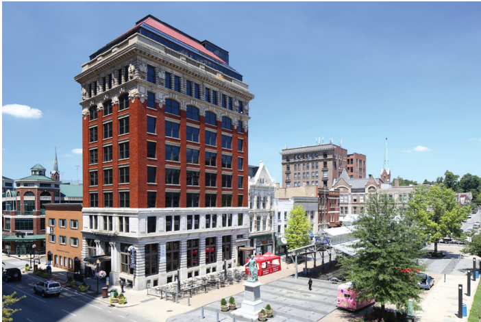
Court Square Building Renovation , Lexington, KY
