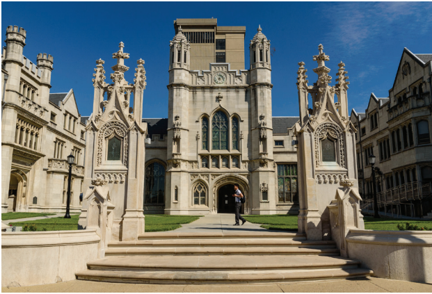
Above: JCTC Seminary Building Stabilization and Renovation
