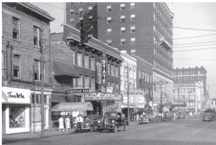
Kentucky Theater and State Theater Renovations , Lexington, KY
