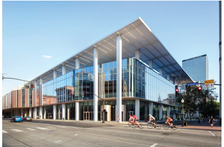
Kentucky International Convention Center Expansion , Louisville, KY
