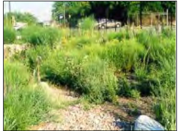
Bio Swale filtration area.
