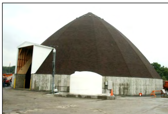
Des Plaines Salt Dome Storage and Deicing Facility.
