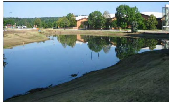
Wet Detention Pond
