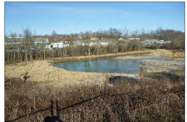
Former lagoon area with randomly placed fill.
