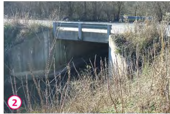
2 Culvert Under Cutters Hill Road
