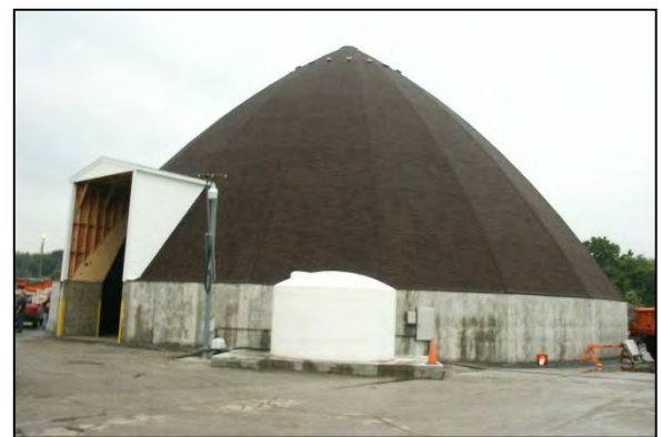
Salt Dome Storage and Deicing Facility.
