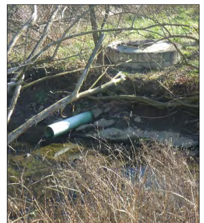
Existing manhole at creek.
