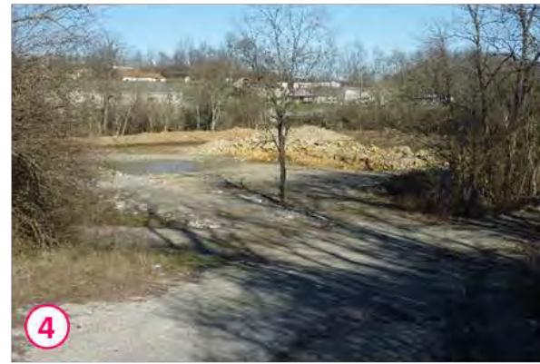
4 Fill Placement in Lagoon
