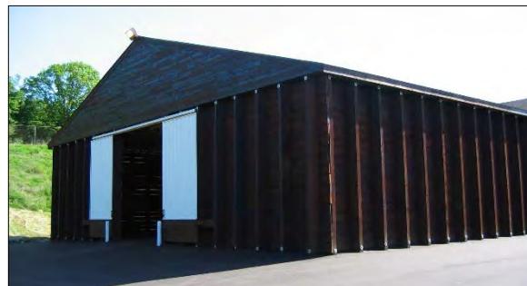
Sand/Salt Storage Facility.
