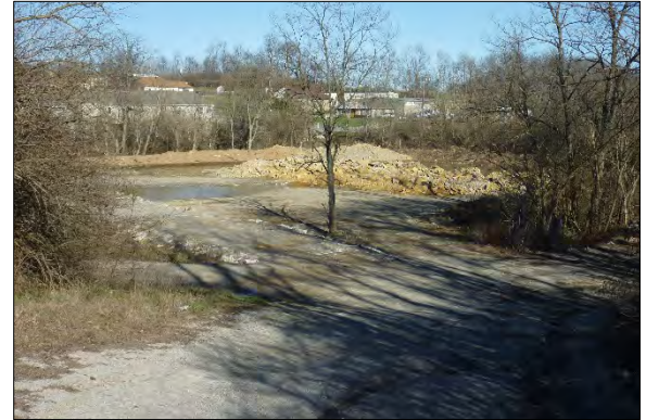
Existing rocky fill to be evaluated for re-use.
