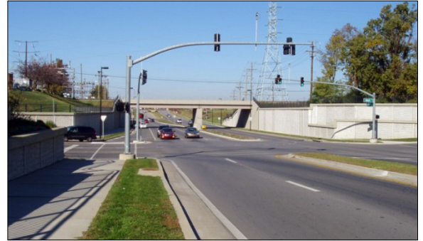
West Reynolds Road Railroad Underpass Reconstruction.
