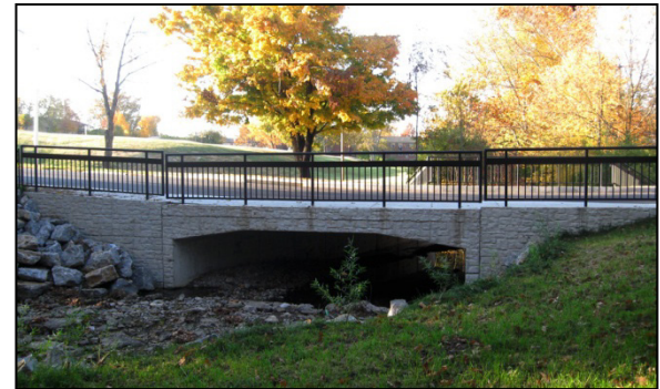
Appomattox Road Bridge/Culvert Replacement.
