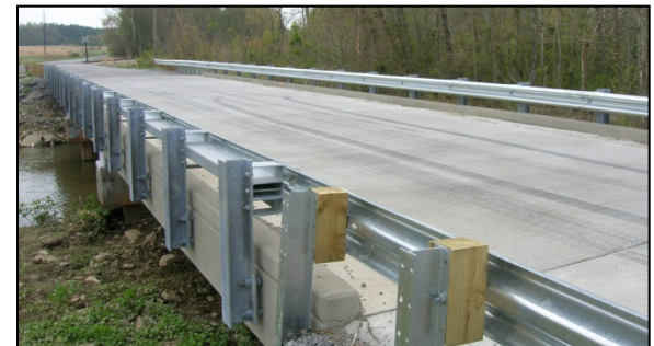
Bean Cemetery Road Bridge Replacement. Madisonville, KY.
