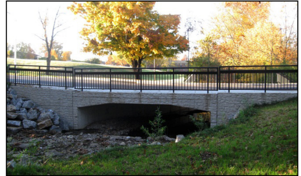
Appomattox Road Culvert Replacement 24-foot x 6-foot R.C. Box Culvert.
