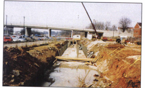
Chambered 12-foot x 6-foot storm and 5-foot x 4-foot sanitary R.C. Box Culvert - Downstream.
