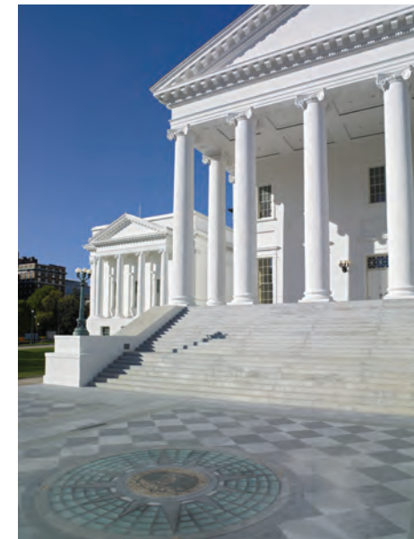
Virginia State Capitol Complex - South Portico
