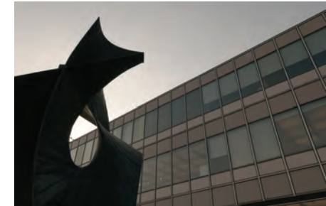
General Motors Technical Center
