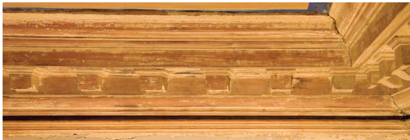
Photograph of 17th-Century Wood Cornice During Paint Removal
