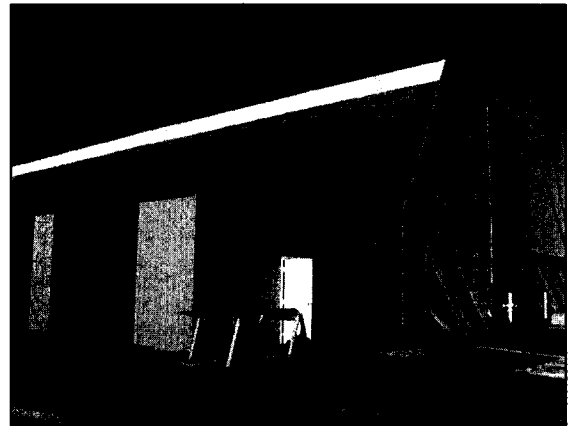
Illinois Tollway Salt Storage Facilities Maintenance Yards M-11 & M-12.
