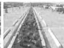
Parking Lot Bioretention
