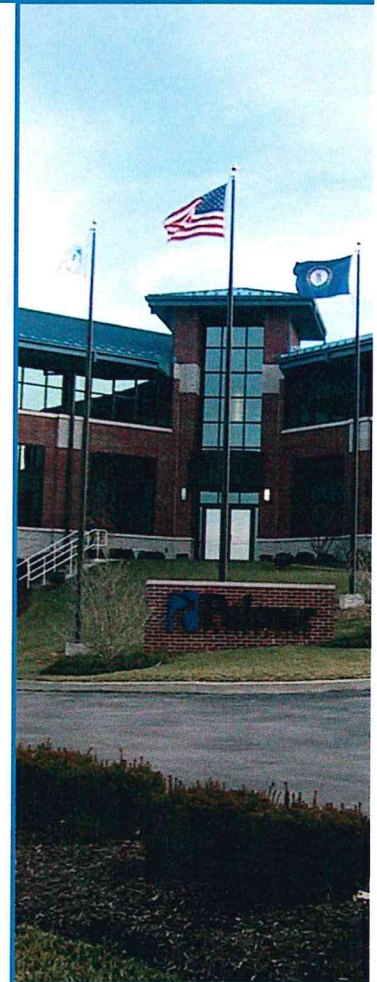
Palmer Engineering Headquarters Winchester, KY
