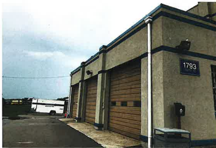
North Façade – Garage Doors
