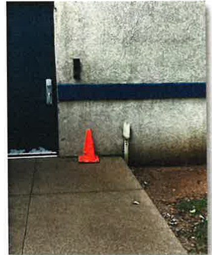
Access Control Device – EIFS at grade
