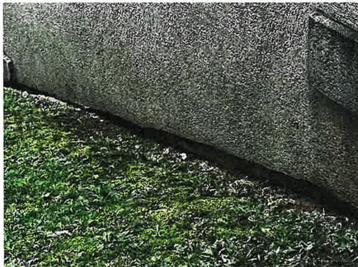
EIFS detail at sloping grade
