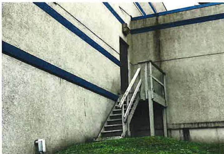
Steel egress stairs from gymnasium
