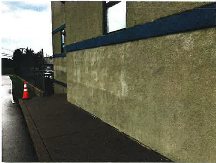
West Roll Call building – West Façade
