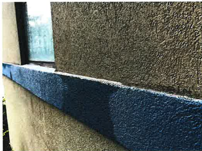
Caulking on horizontal bands to repair cracks in EIFS
