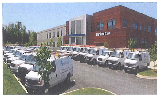
Harshaw Trane, Louisville Headquarters
