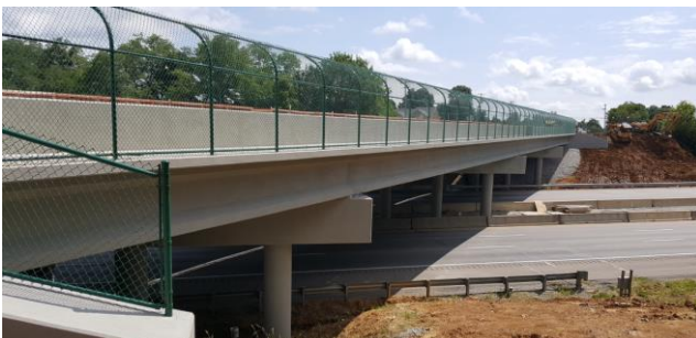
Recently constructed Andover Country Club golf cart tunnel (top) and bridge over I-75.
