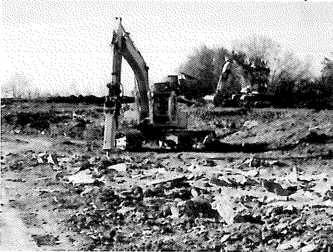
PHOTO 1- HITACHI HOE RAM USED TO BREAK UP BOULDERS PHOTO 2- 2 MINUS ROCK USED FOR HAUL ROADS
