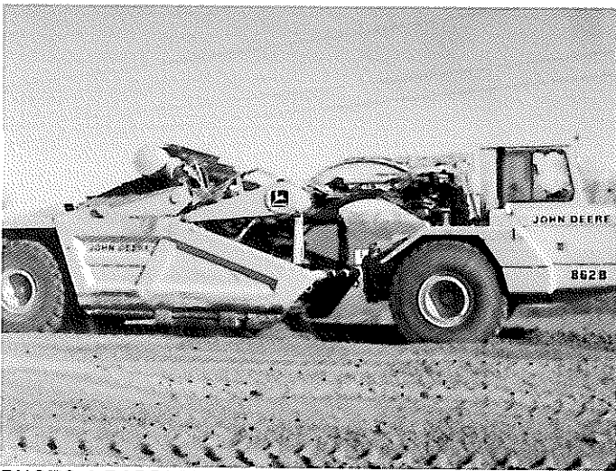
PHOTO 1-PADDLEWHEEL SCRAPERS STOCKPILE SOIL
