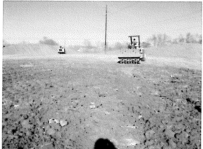
PHOTO 2- SHEEPSFOOT PULVERIZES ROCK PARTICLES
