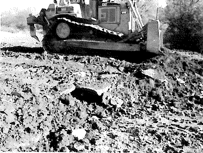
PHOTO 1- CATERPILAR D6 BULLDOZER GRADES FILL
