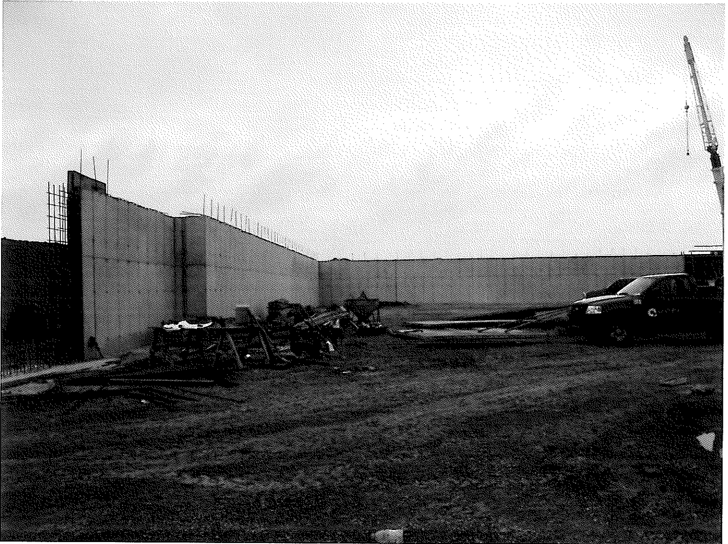
AREA A / AREA B RETAINING WALL FACE WHICH DOES NOT DISPLAY HONEYCOMBING, CRACKING, OR FINS
