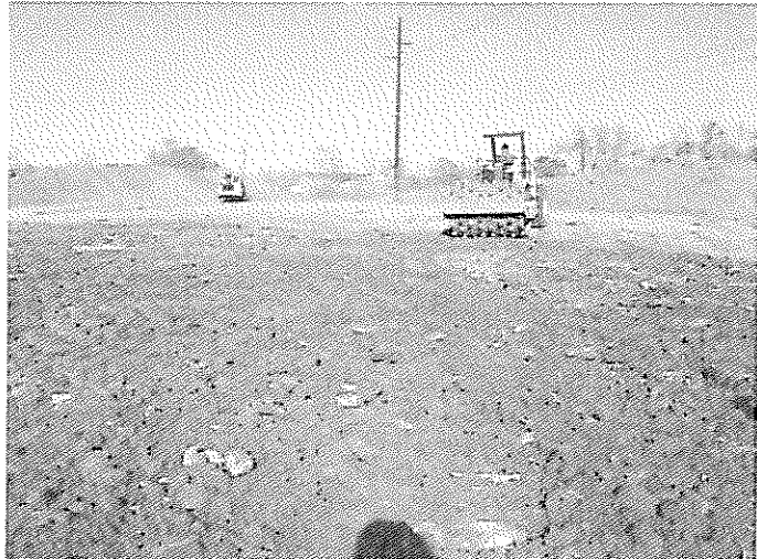
PHOTO 2- SHEEPSFOOT PULVERIZES ROCK PARTICLES
