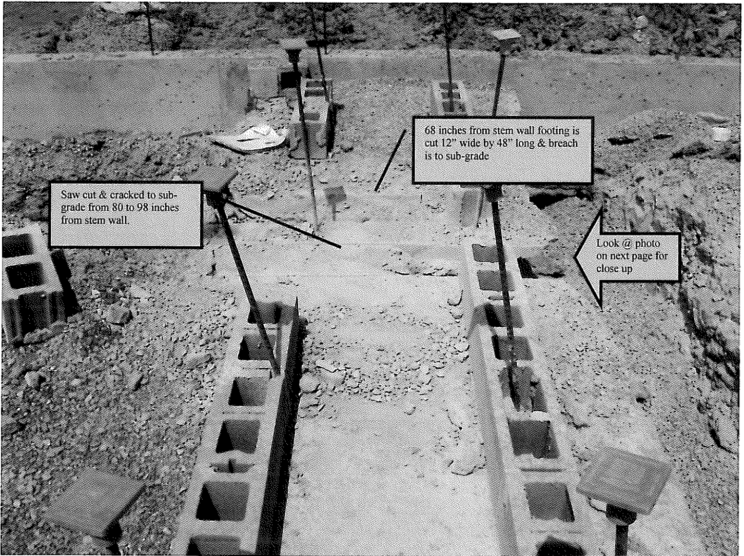
ARROW SHOWS BREACHES IN AREA A CHASE @ BOYS AND GIRLS RESTROOM 116 AND 117
