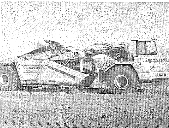
PHOTO 1-PADDLEWHEEL SCRAPERS STOCKPILE SOIL
