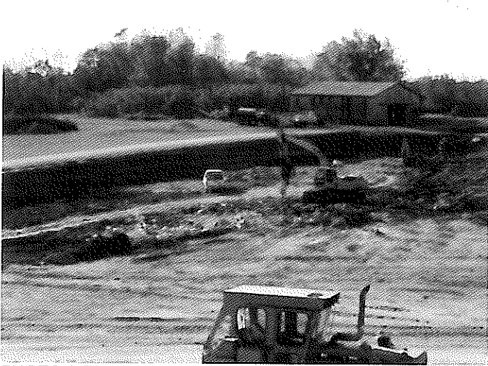
PHOTO 3-BUILDING PAD LOOKING NORTH
