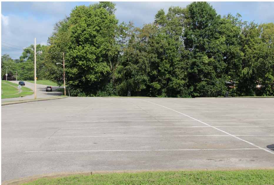
FIGURE #1: existing conditions for the larger asphalt Southland Park Parking Lot
