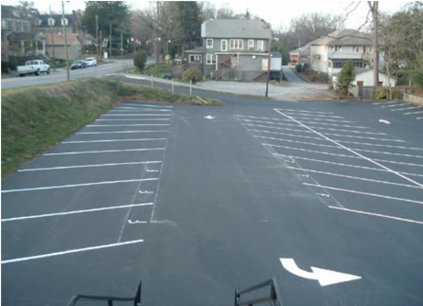
FIGURE #6: example of a one-way two-sided parking lot striped at a 45° angle with the correct pavement width
