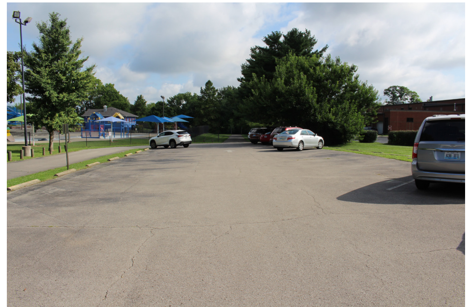
FIGURE #2: existing conditions for the smaller asphalt Southland Park Parking Lot
