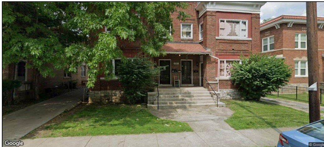
271 East Maxwell Stret - 2-story, wire brick Arts and Crafts fourplex. Two story porch. flanking entrance bay have been filled in. Parapet in center bay has decorative brick panel. Red tile overhang on entrance. Apartments in 1927.
