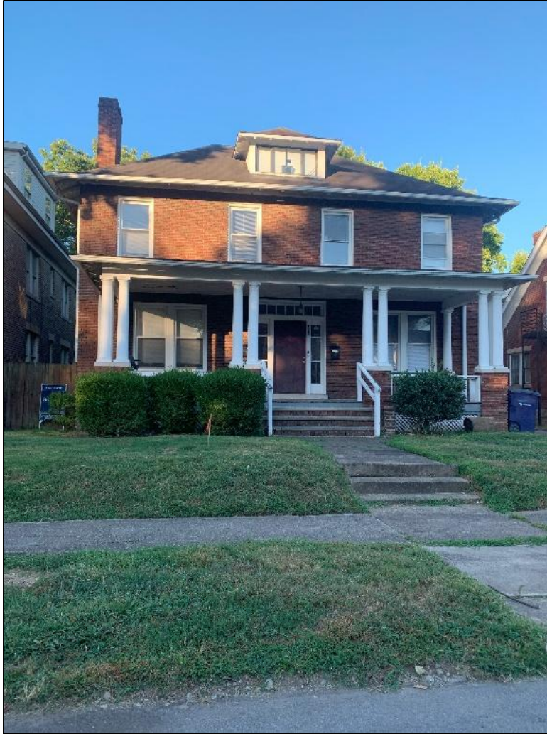
268 - 2-story, three-bay, brick Arts and Crafts house with double window dormer projecting. One-story porch has Tuscan columns. 1921 - Joseph Levy.
