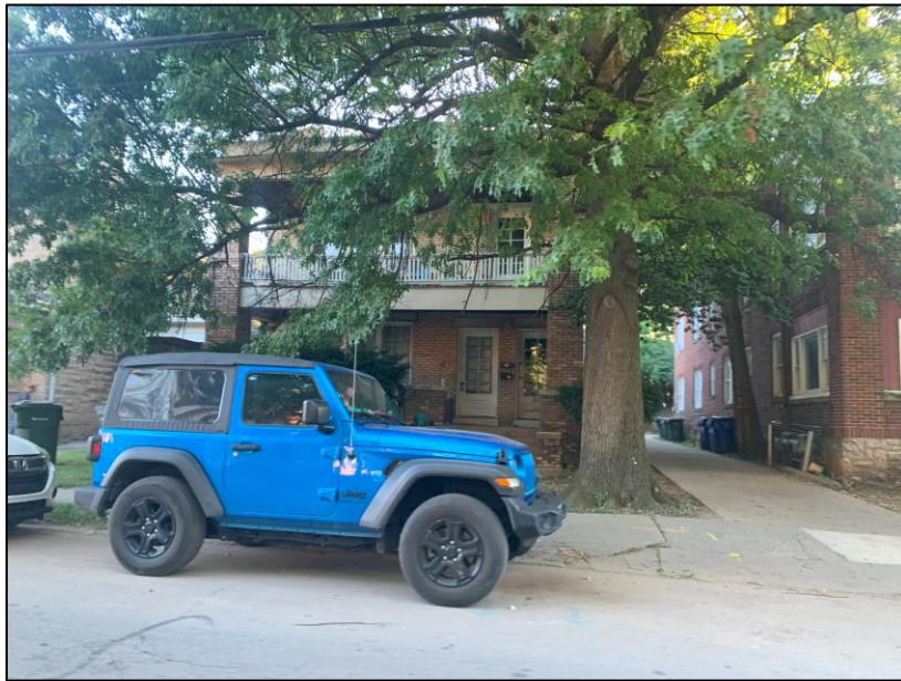
261-63 East Maxwell Street- 2-story, 2-bay tan brick Arts and Crafts/Colonial Revival duplex. Two-story gallery porch on front facade has square brick piers. 1927 - J.F. Wise at 261, W.P. Fishback at 263.
