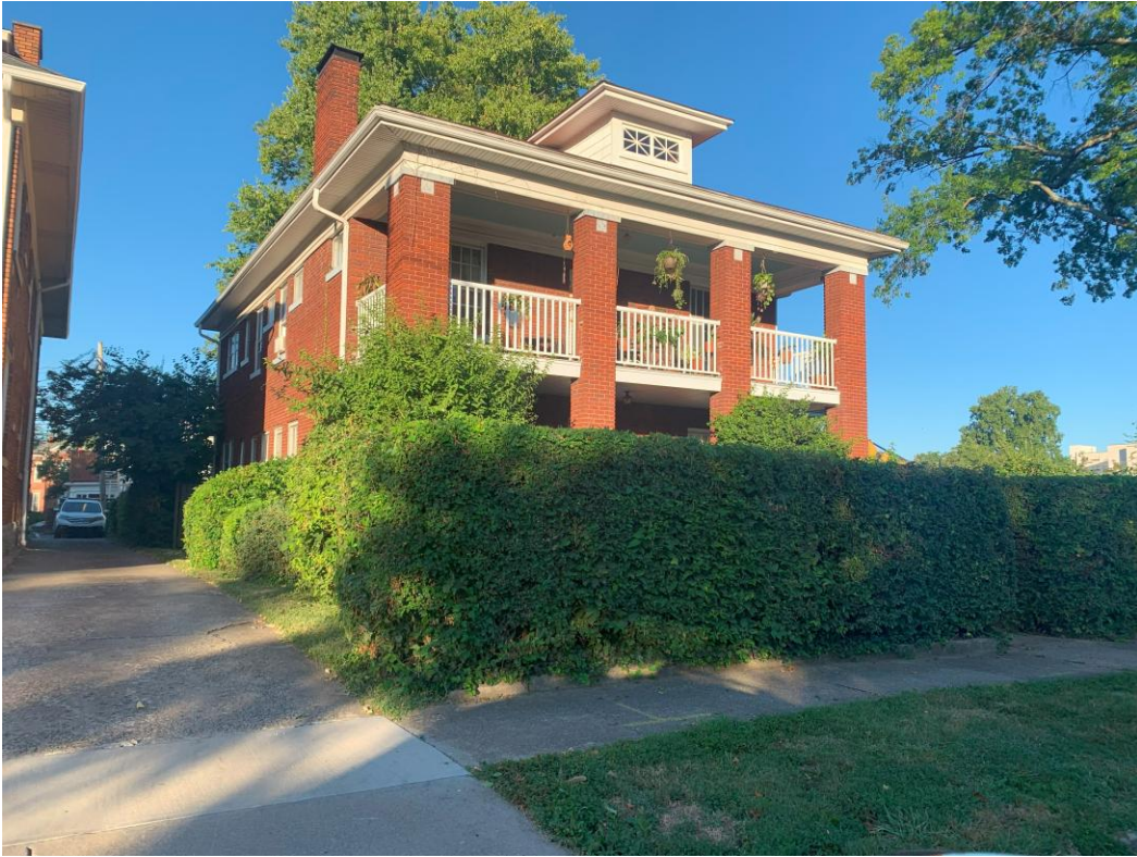
256 Kalmia- 2-story, three-bay, brick Arts and Crafts duplex with red tile roof intact. Two-story porch, large brick piers. 1923 associated with Samuel Bederman.
