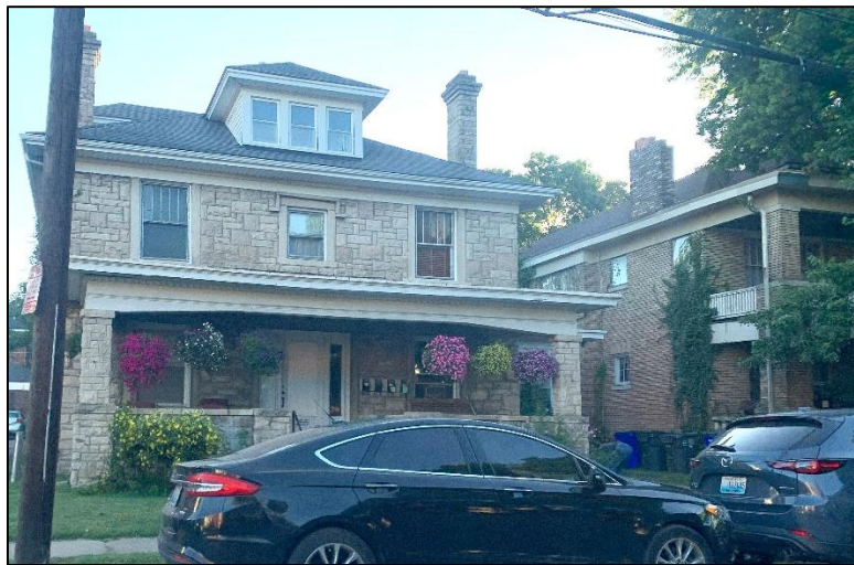
255 East Maxwell Street – 2-story, rectangular stone, Arts and Crafts house with full one-story porch. The structure has triple window, hipped roof dormers on front and sides. Chimneys are corbeled. Built circa 1915 by Richard Spurr Webb, Jr. and his wife Allie. Possible designed by Frankel and Curtis. This is the most significant structure on the street.
