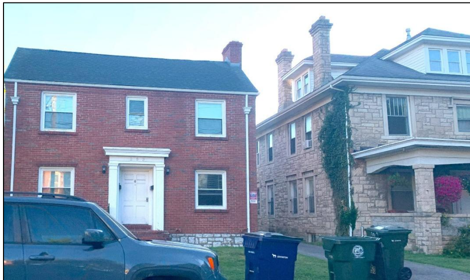
253 East Maxwell Street- 2-story- 3-bay, Colonial Revival brick structure with engaged chimney on one side. The structure, built in 1929, has a stone foundation and later built two story brick addition.
