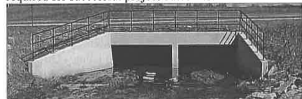
Wellington Development Box Culvert – Lexington, KY.
