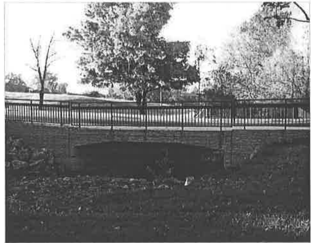
Appomattox Road Culvert Replacement - Double 12-foot x 6-foot R.C. Box Culvert.
