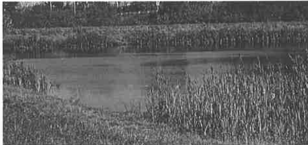
Ellerslie Regional Detention/Water Quality Basin (Expansion Area 2C - Basin C4) – Lexington, KY.
