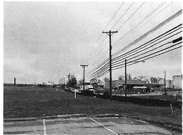
Overhead utilities along Old Frankfort Pike.
