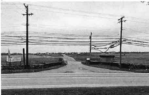
Existing overhead utilities along Old Frankfort Pike.
