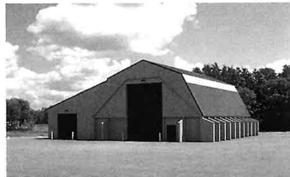
USH 41 salt shed in Ashwaubenton, Wisconsin.
