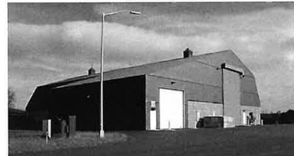
Dane County salt shed designed as part of the Verona Road project.
