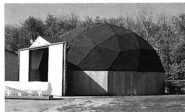
Fontana's salt storage building.
