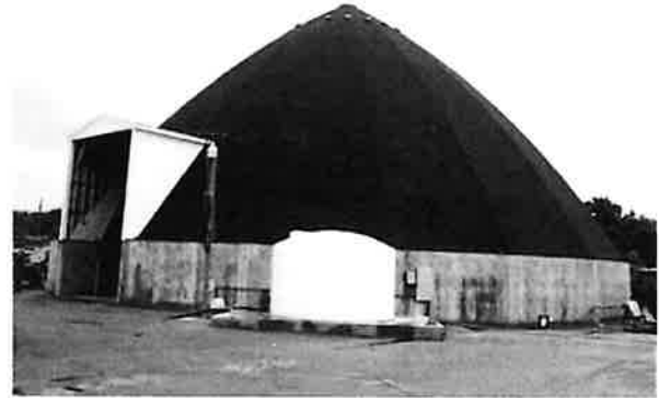
Salt dome storage and deicing facility, Des Plaines, IL.
