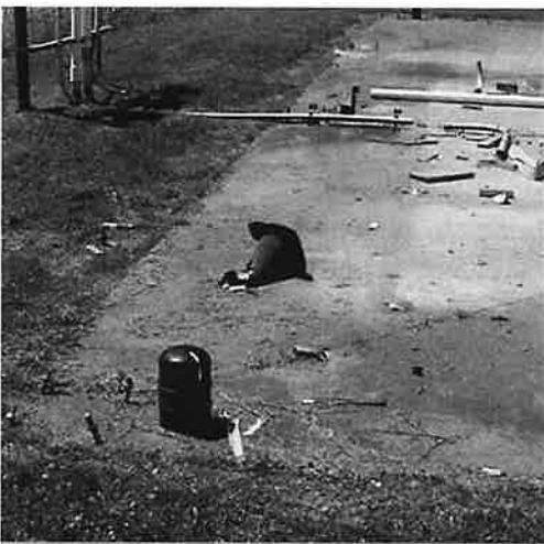
Figure 4.2: Landfill Gas Management System Vent
