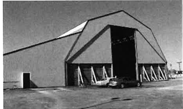
Illinois Tollway's new salt storage facility.
