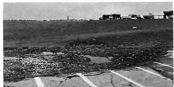
Steep slopes adjacent to existing building pad.
