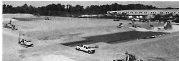
Special Geogrid reinforced pavement section for construction traffic loading. (10/17/16)
