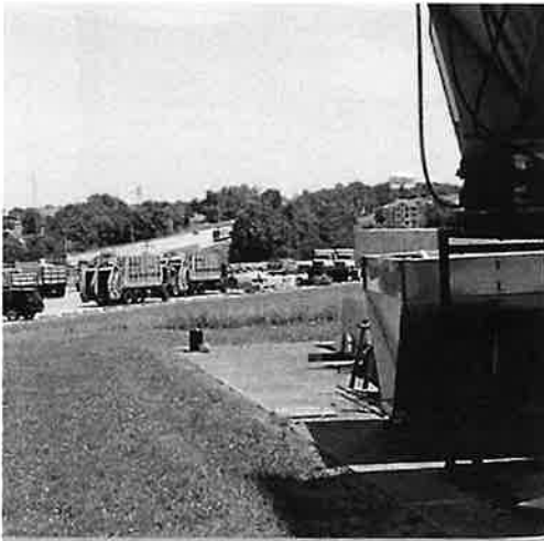
Figure 4.1: Landfill Gas Management System Vent
