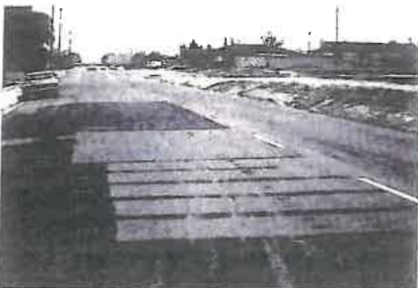
Reclamite was used as a construction seal on the dry areas of the pavement.
