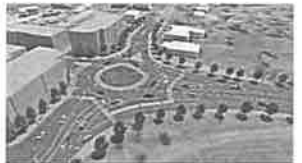
Reagan Expressway Terminal -Gateway Roundabout Intersection
