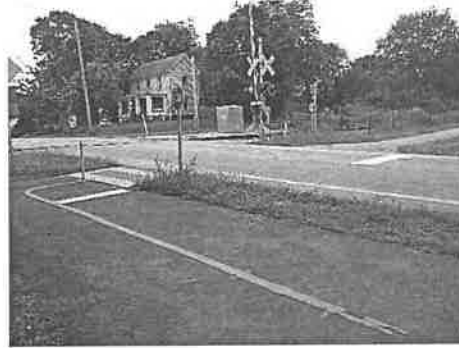
Existing railroad crossing at Mound Street.
