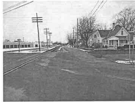
Existing railroad crossing at Mound Street.
