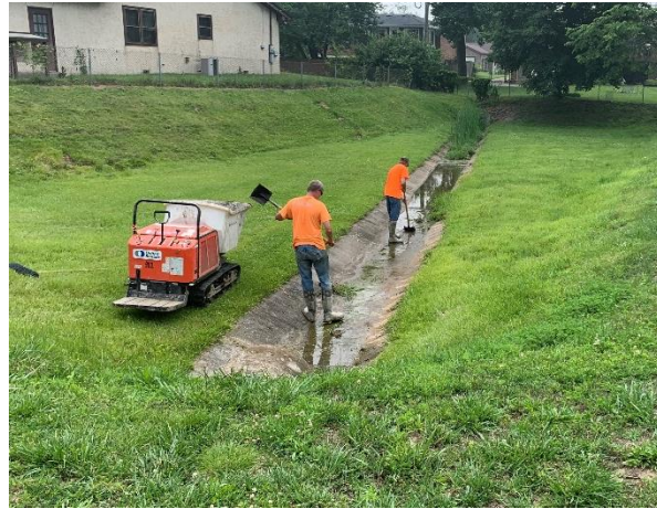
Cleaning Concrete Flumes
