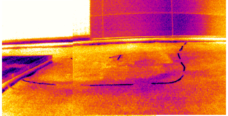
Infrared view of area #
