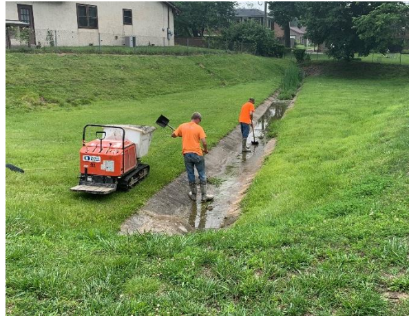
Cleaning Concrete Flumes
