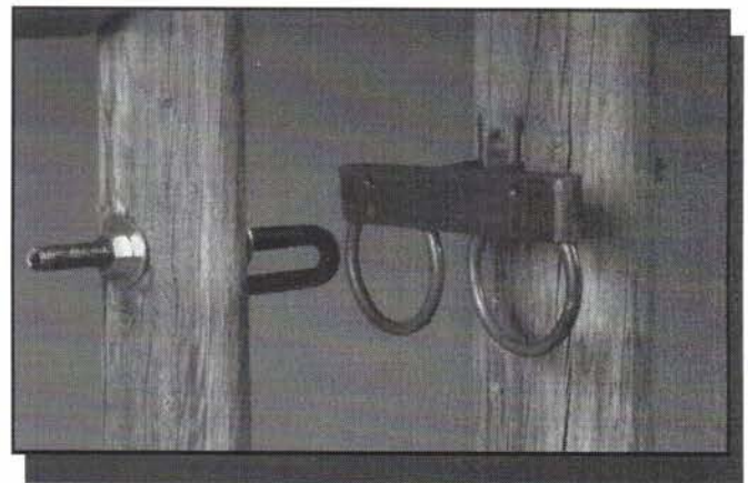
Figure 1—The original ring latch manufactured by the Hamilton Hinge Co.
