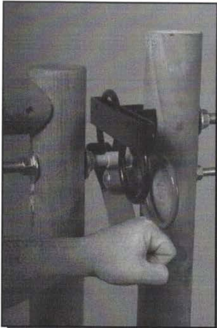
Figure 4—One hand presses down on the lever (green) of the accessible latch.
